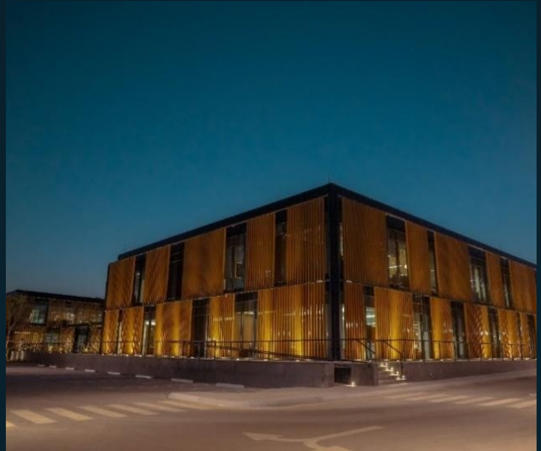
ROSHN OFFICE BUILDING / SEDRA 2, RIYADH
